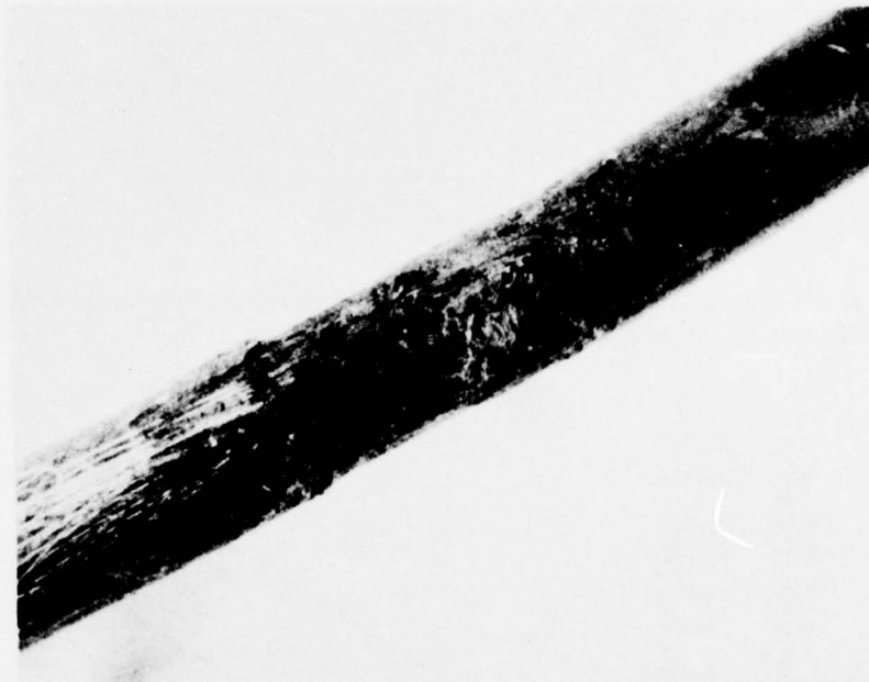
Figure 17. Localized corrosion attack in the copper cladding after 15 months exposure in brackish water. (Block 48)
