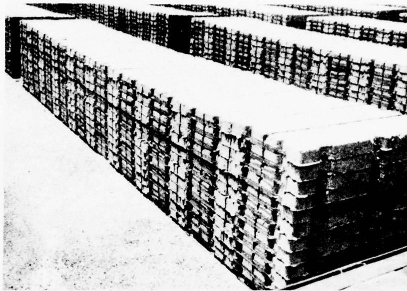
Figure 2. "Squares" after casting. The squares consist of concrete slabs cast onto the wire fabric.
