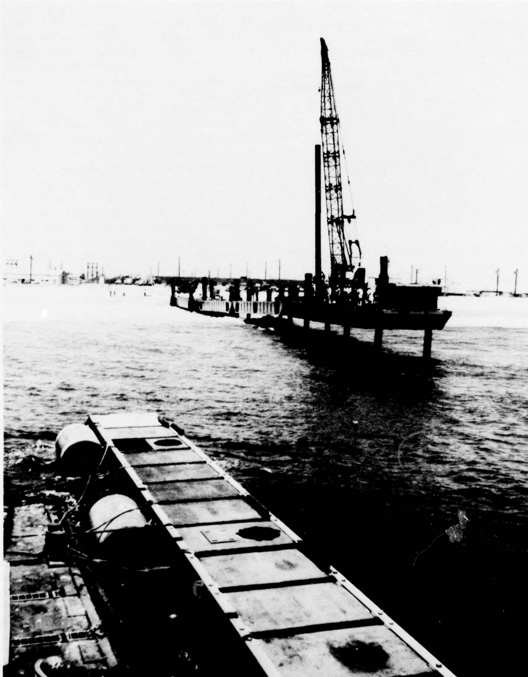
Figure 1-5. Fender unit approaching elevated pier. Note 50-foot (15.2-m) piles ready for dropping into center spudwell of fender unit.
