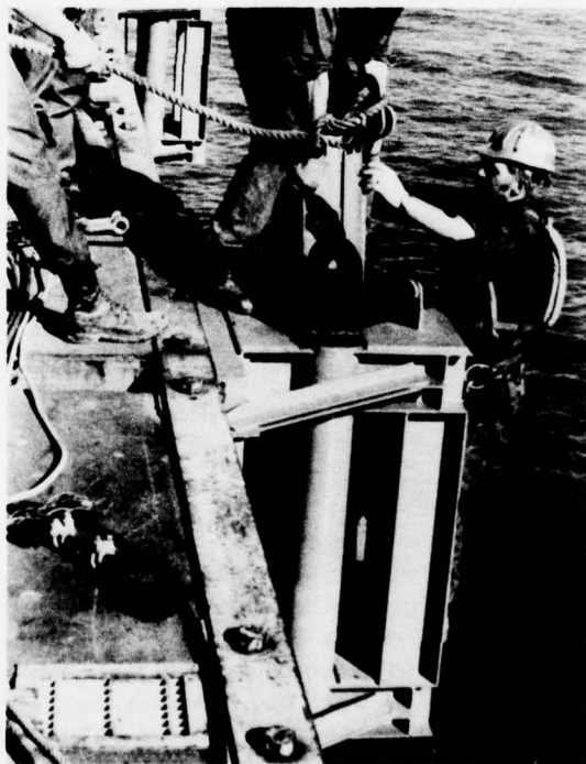
Figure 1-10. Installing pile guide in external spudwell.
