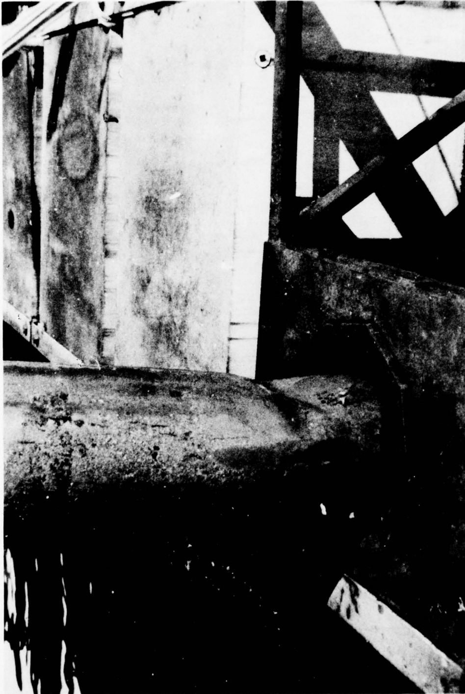
Figure 1-21. Failed fender pile.
