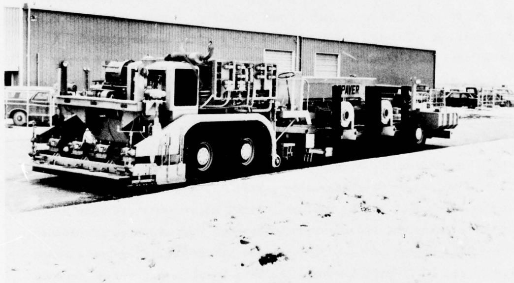
Figure 6. Bituminous pavement repaver
