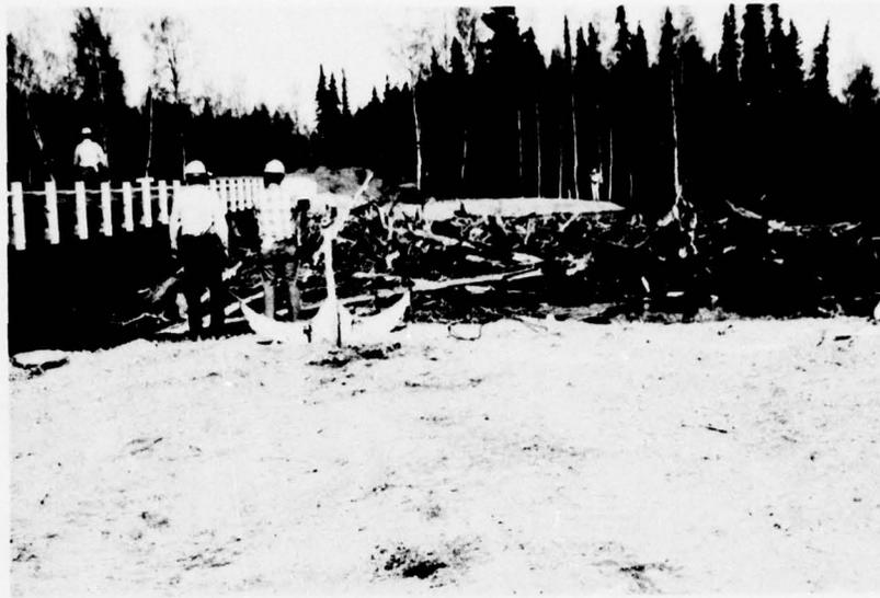
*Figure 4. Debris accumulation behind bridge at damsite (12 May 1975). Note trash hook in foreground.*
