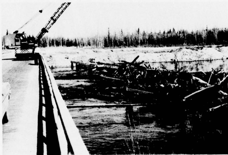
*Figure 5. Debris accumulation on trash racks at Engineer Bridge, Fort Wainwright (12 May 1975). Note that debris did not accumulate against the bridge pilings.*
