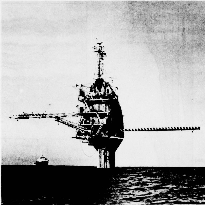
Fig. 1. Research Platform FLIP with temperature profiling array.
