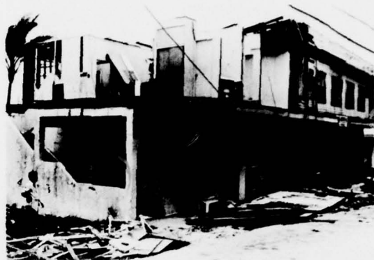
FIGURE 4-11. Destruction was widespread in Guam's civilian community. Concrete structures fared well, but wooden houses, power lines and the telephone system were all severely damaged. (Official U. S. Navy photograph)
