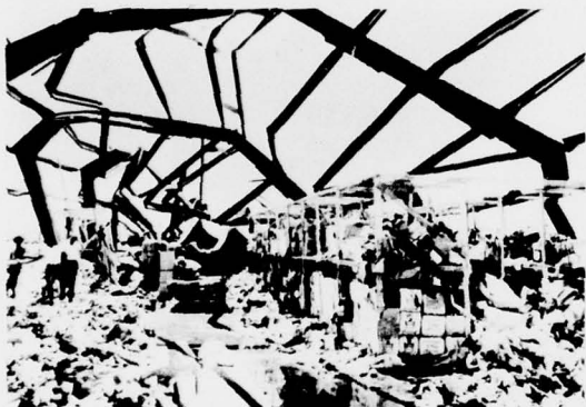
FIGURE 4-10. The twisted steel skeleton of a once substantial warehouse attests to the destructive force of Pamela. (Official U. S. Navy photograph)
