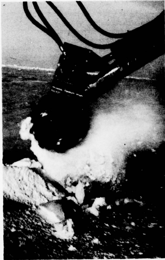
Figure 17. Removing ice hummock with ice chipping drum attached to backhoe arm.
