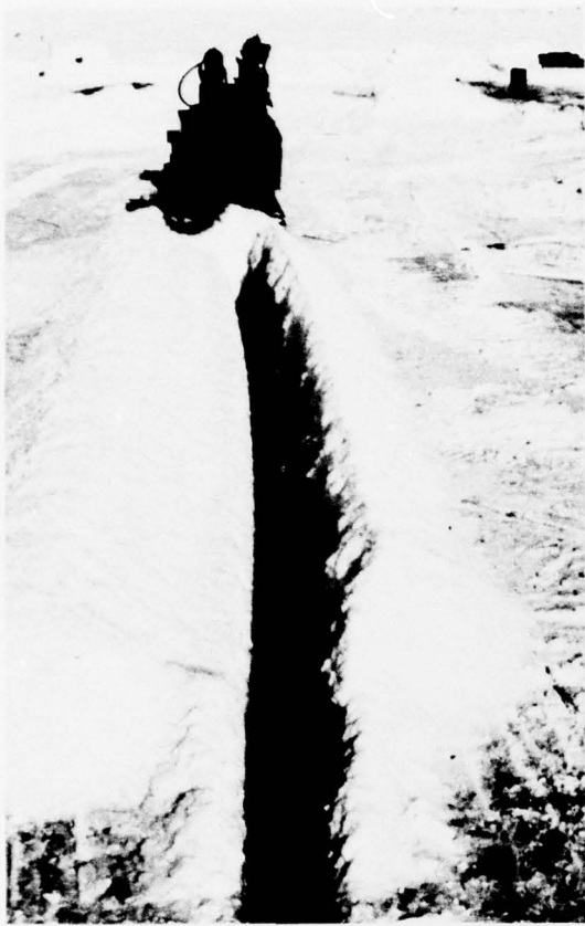
Figure 15. Part-through trench in 78-inch (200-cm) thick ice sheet showing gradual curve to left.
