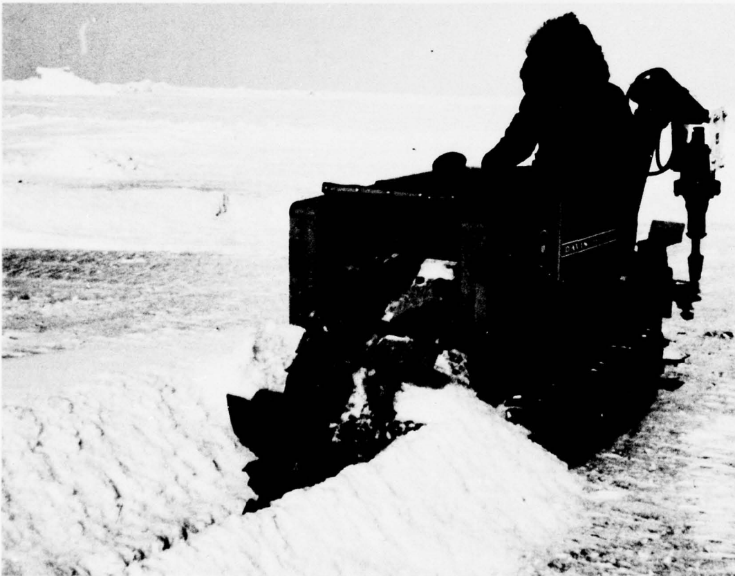
Figure 14. Ice excavation machine performing trenching operation, cutting 60-inch (150-cm) trench in 78-inch (200-cm) thick ice sheet.
