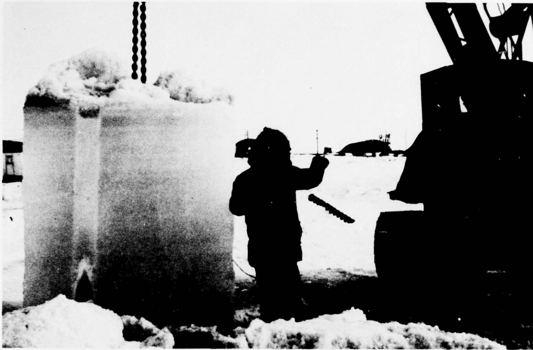
Figure A-2. Ice block showing refrozen trench being hoisted from ice sheet.
