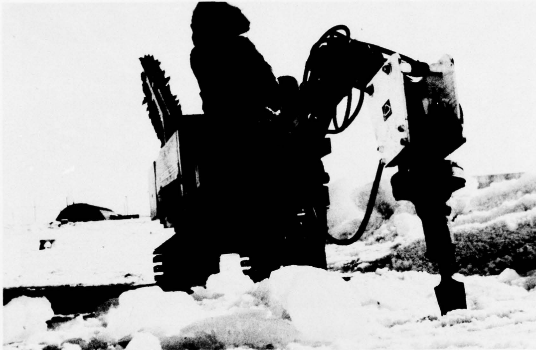
Figure 18. Impactor attachment with frost spade working tool excavating anchor pit on ice sheet surface.
