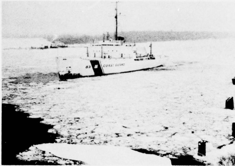
*Figure 2. Ferry-stopping ice being cleared by U.S. Coast Guard icebreaker.*
