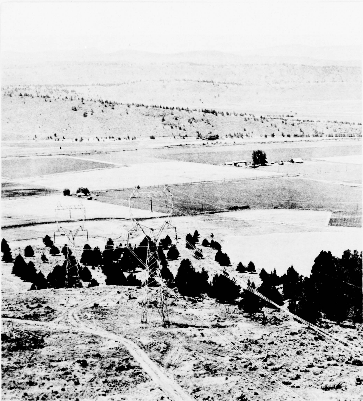
Photo V-1. 500-kv Transmission Line Crossing Farm (USBPA Photo).
