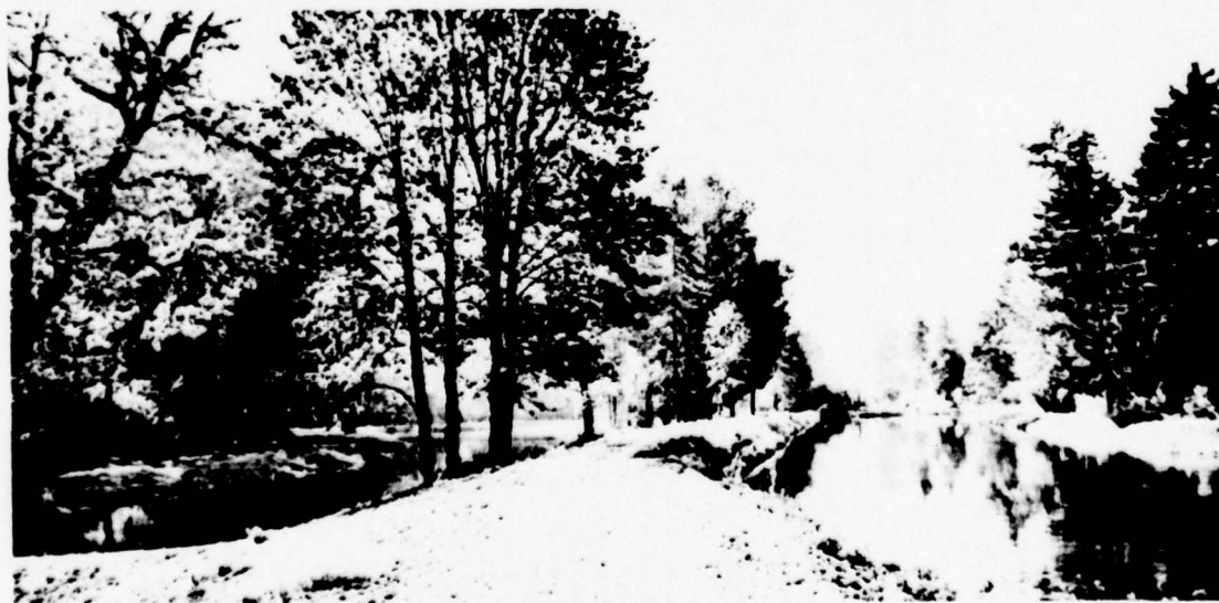
Photo II-6. Infiltration galleries. City of Salem water supply system on Stayton Island. (City of Salem, Municipal Water Works Photo)
