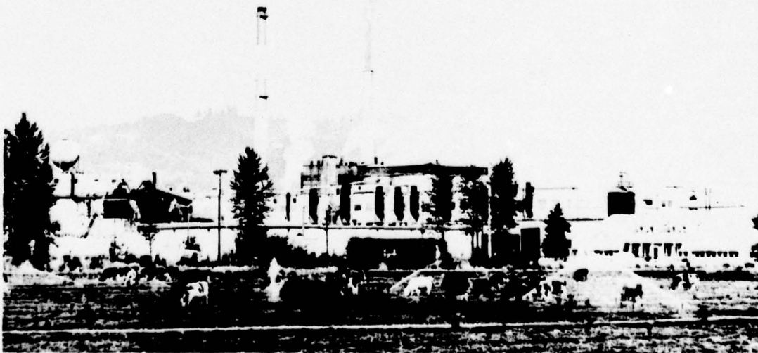
Photo II-2. The Weyerhaeuser plant in Springfield is the major industrial water user in the Upper Subarea.
