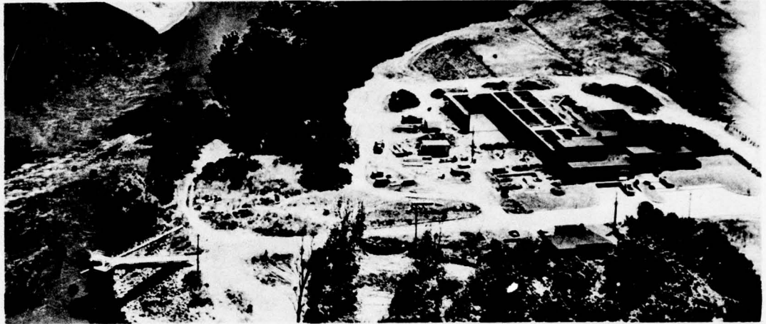
Photo IV-1. Willamette River water is withdrawn and treated here before use by the people of Corvallis during summer low-flow months. (Cornell, Howland, Hayes and Merryfield, Corvallis, Oregon, Photo)
