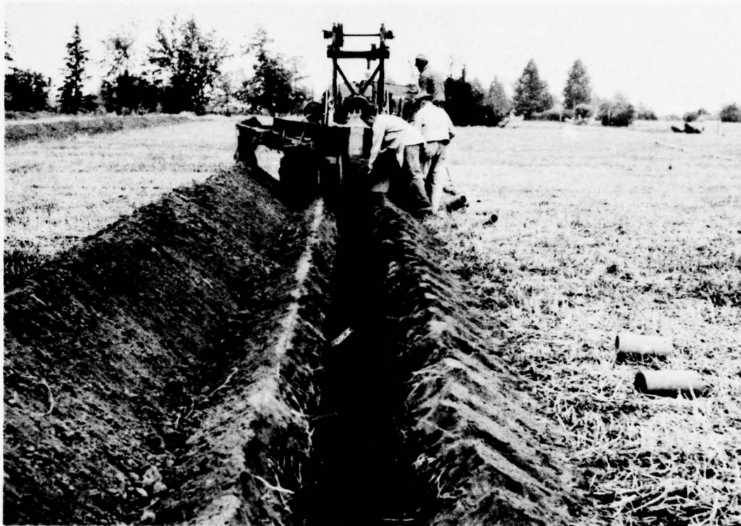
Photo IV-3. Tile laid in trenches may be needed to drain fields where the water table is near the surface.
