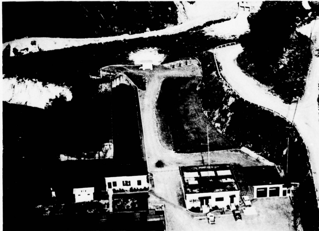
Photo IV-10 Water from Bull Run River is diverted at the headworks for Portland's municipal supply.
