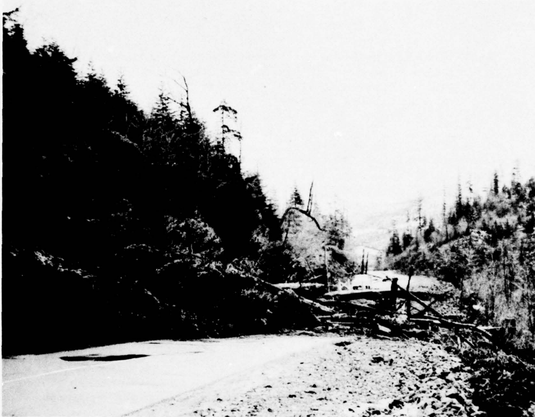
Photo IV-2. Landslides, such as this one during the December 1964 flood, are major contributors to sediment load in Willamette Basin.
