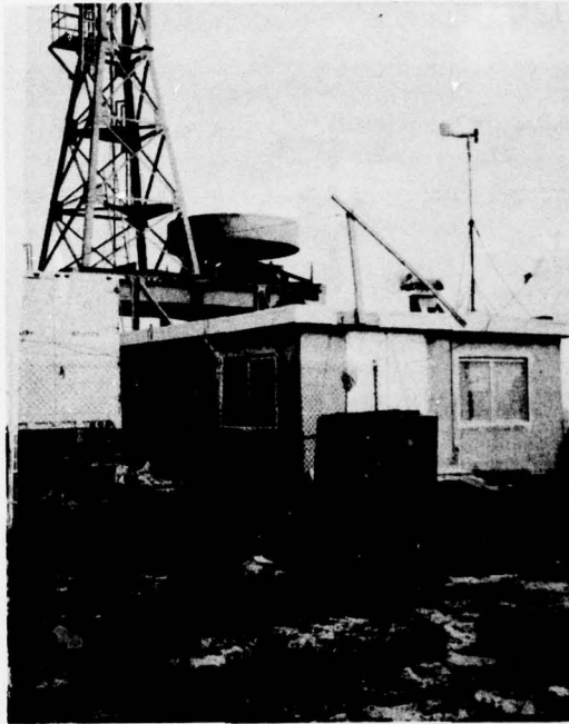
Fig. 8 - South end of south building
