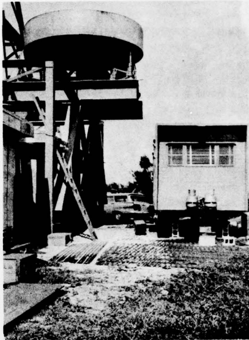
Fig. 12 - Lower section of tower, east side
