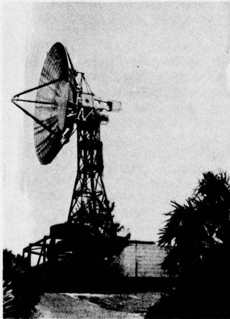
Fig. 15 - Full view of tower, west side
