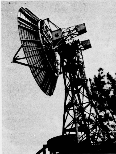
Fig. 14 - Center and upper sections of tower
