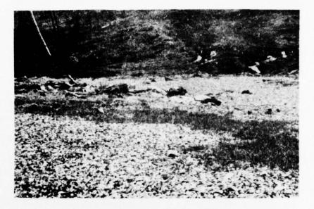
Figure 25. Chips placed on steep slope of relocated state highway.
