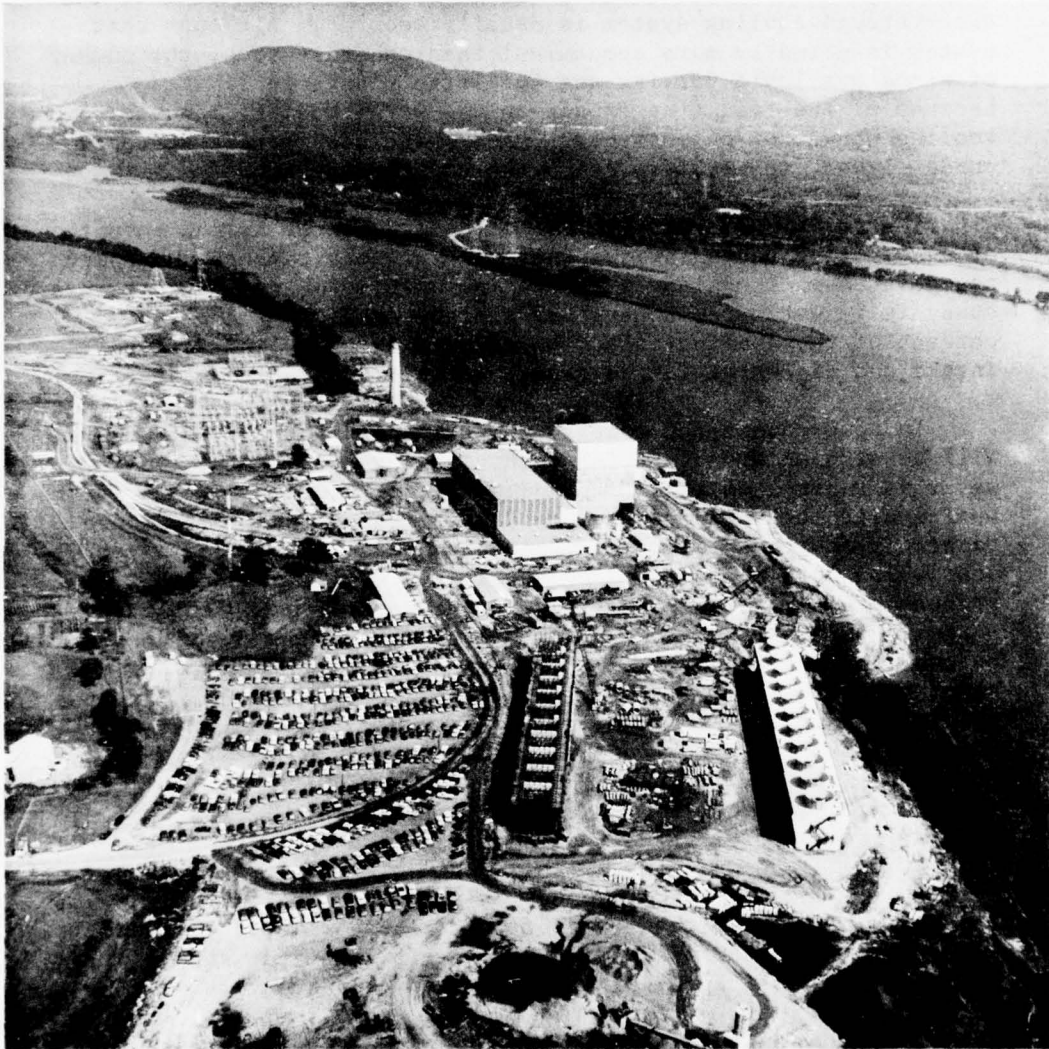
Vermont Yankee Nuclear Station under construction, showing the partially completed mechanical draft evaporative cooling towers (wet).
