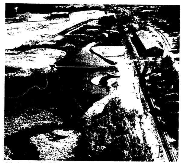
This "morning glory" intake conveys flood waters to an underground conduit at Wordester, "assachusetts. (Department of the Army, New England Division, Corps of Engineers).
