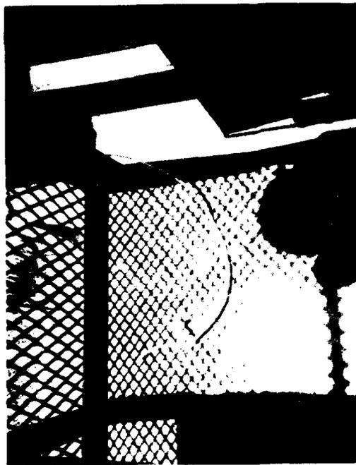
**Figure 6.** In an actual installation it is often easy to circumvent the integrity of a protective enclosure. In this example, a communications cable brings a ground into the enclosure.
