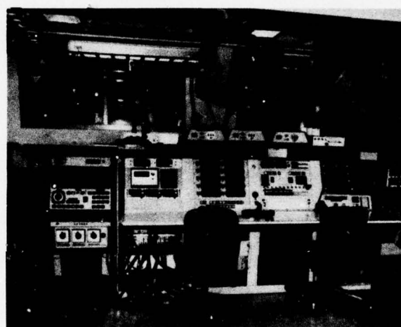
Fig. 8 Operator's control console.
