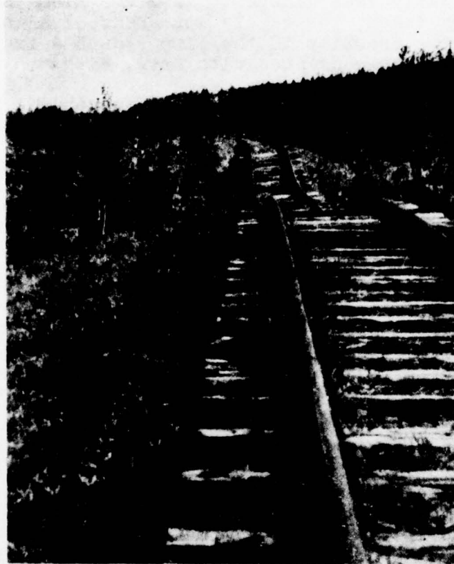
Figure 7. Section of unused railway east of Salekhard. The disturbance of heat exchange in the permafrost led to melting of the subsurface ice under the roadbed and its settling. (Photograph by A.I. Dement'yev.)
