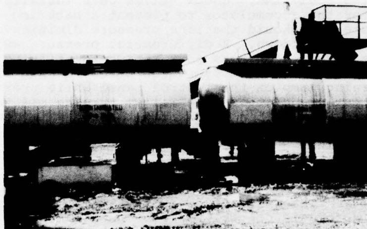
Figure 8. Storage Vessels - Seymour Johnson AFB
