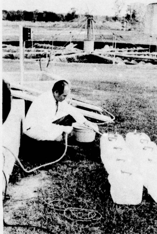
FIGURE 11.--Collection of Settled Primary Domestic Sewage. This photograph illustrates the delivery of settled primary domestic sewage into plastic containers used for transporting the sewage to the laboratory.
