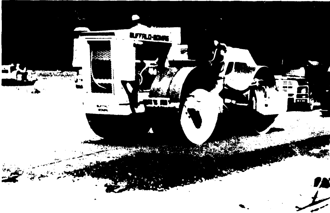
Photo 5. Rolling pattern with vibratory rollers
