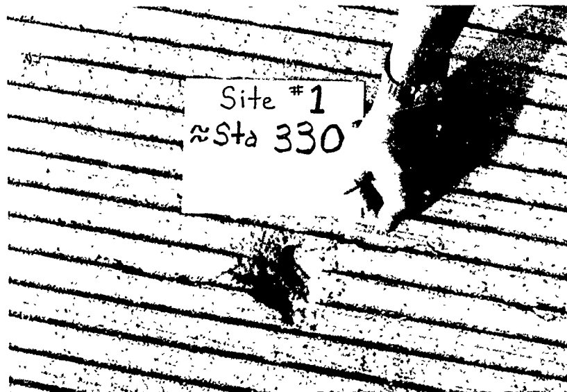
Figure 25. Close-up of an aggregate popout with some distress developing around popout.
