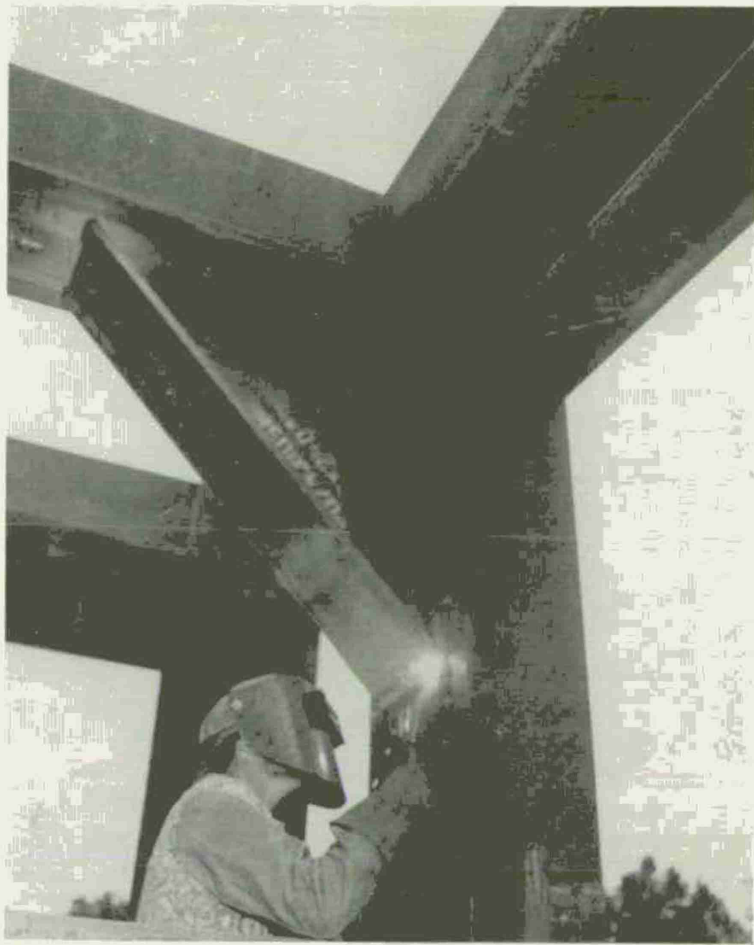
Figure 11. Category 3 Test B3-2 Proof Pressure Test - New Phase II Design Gusset Installation
