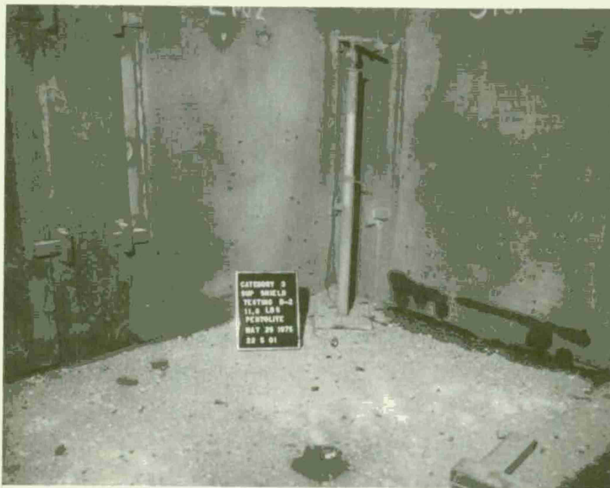
Figure 28. Category 3, Test B2-1, Typical Fragment Damage to Concrete Floor
