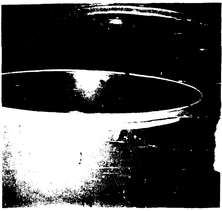
Figure 6. Multi-Seal Gasket on Drum Chime
