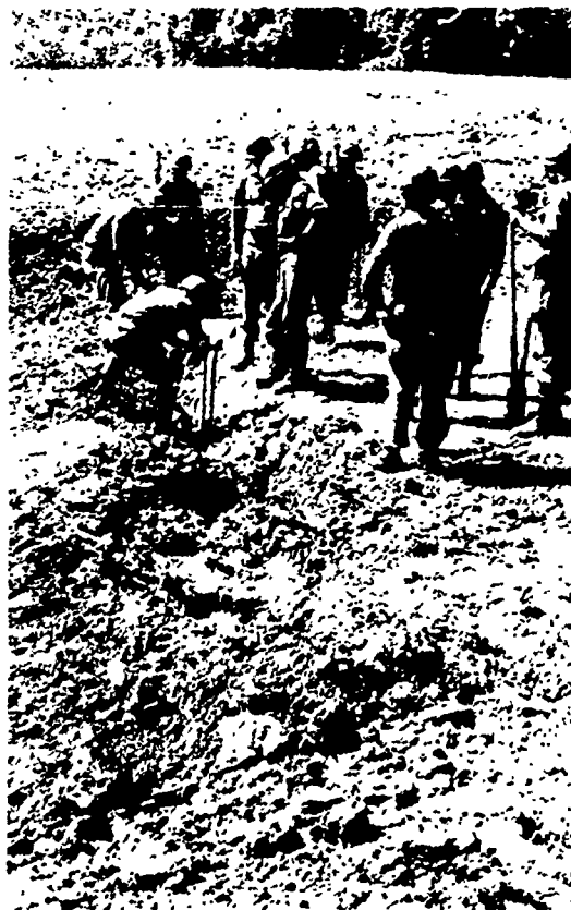
Figure A3. Posthole diggers being used to excavate emplacement holes
