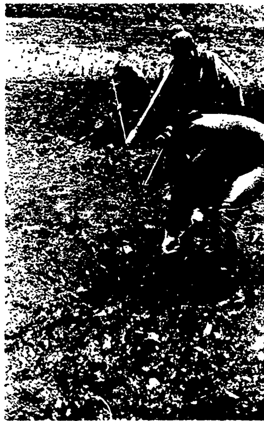
Figure A4. Posthole digger and hand auger being used to excavate slant holes of design G
