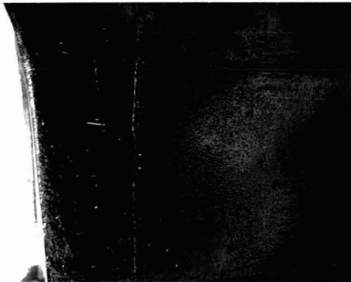
After coal tar epoxy high build coat
