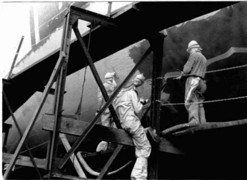
Figure II-16 Photographs Showing the Application of the First Coat of Nonsolvented Polyurethane. This coating was applied and then squeegeed down to fill the pits on the hull of the ship. Subsequent coatings were applied to build up the coating and obtain coverage.
