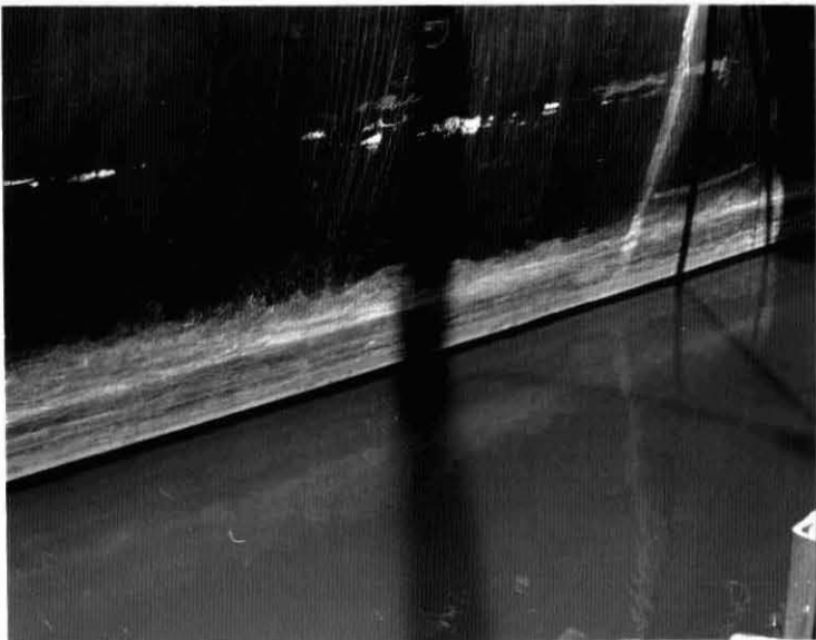
Figure II-24 Typical Appearance of the Polyester Glass Flake Coating at the Waterline on the Hull of the USCG Cutter Westwind (Midship to Stern)
