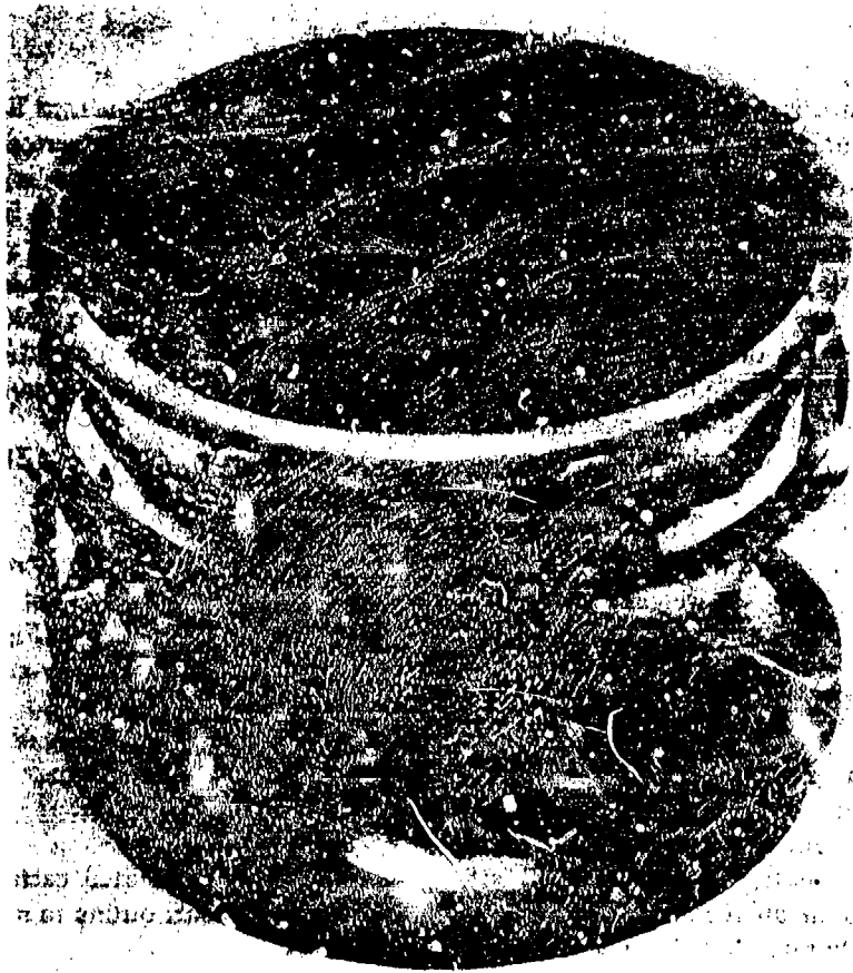
Figure 10-3. Central Expanding Nozzle
