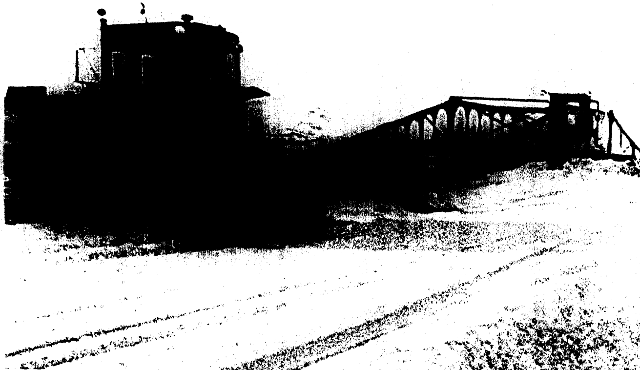
Figure 9. Tractor-towed, 80-foot snow plane leveling previously deposited snow.
