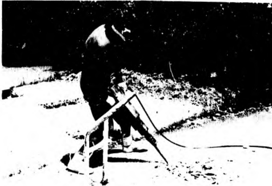
Figure 3. Preparation of Damaged Area
