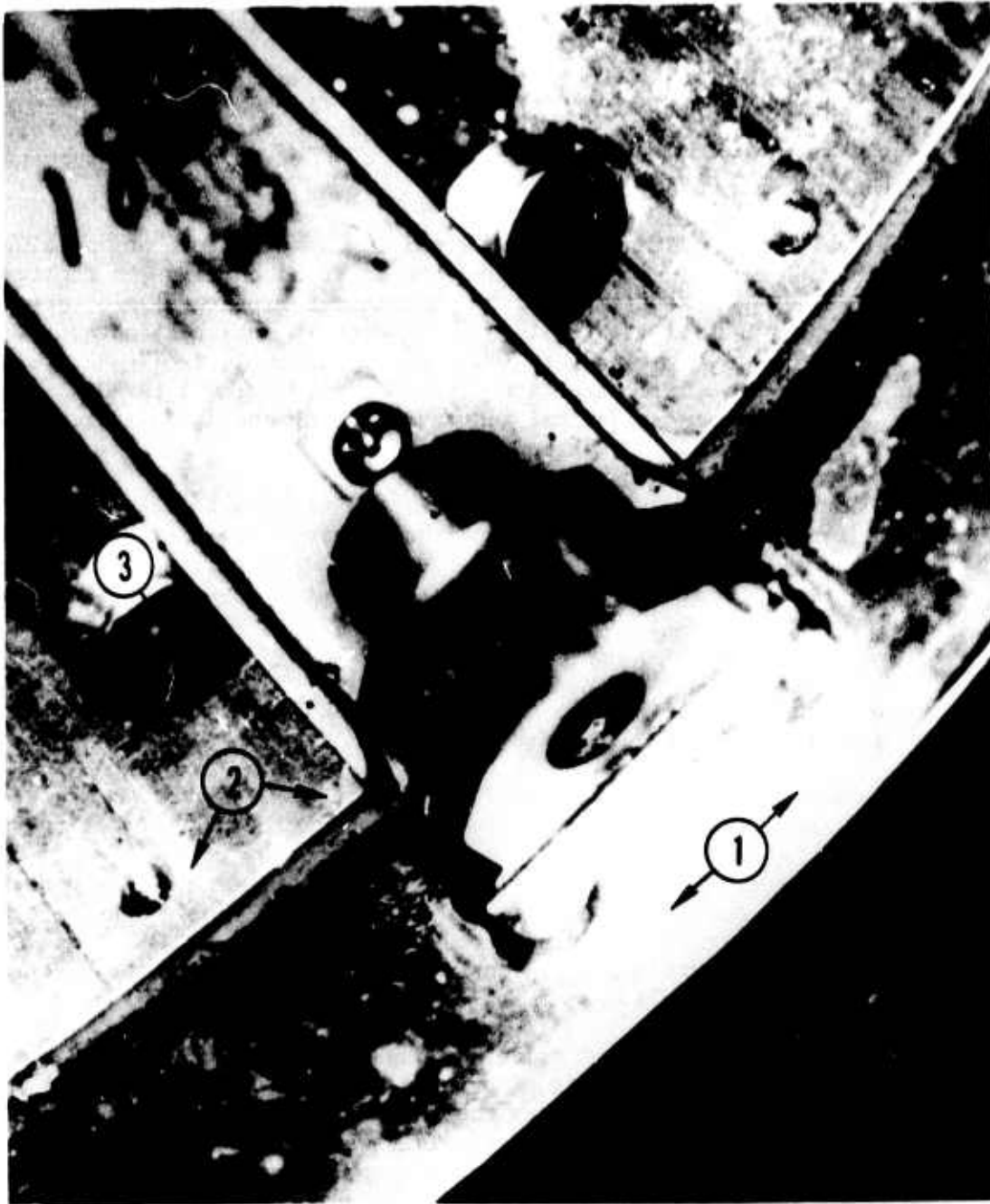
FIGURE 3 - Crevice corrosion, pitting attack, general corrosion, and galvanic corrosion of inside ECM pod structure.
