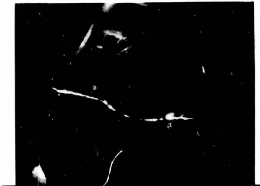
FLORESCENT DYE INDICATION SHOWING CRACK LOCATION
