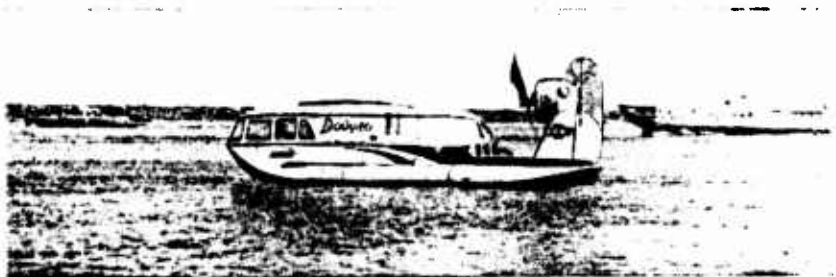
Fig. 19. Raduga Experimental ACV (before addition of flexible skirt) [4].
