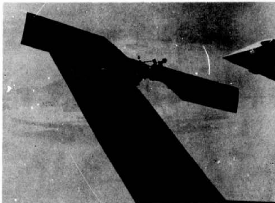
Photo 7. Model 212 Tail Rotor Installation on the YAH-1R Helicopter.
