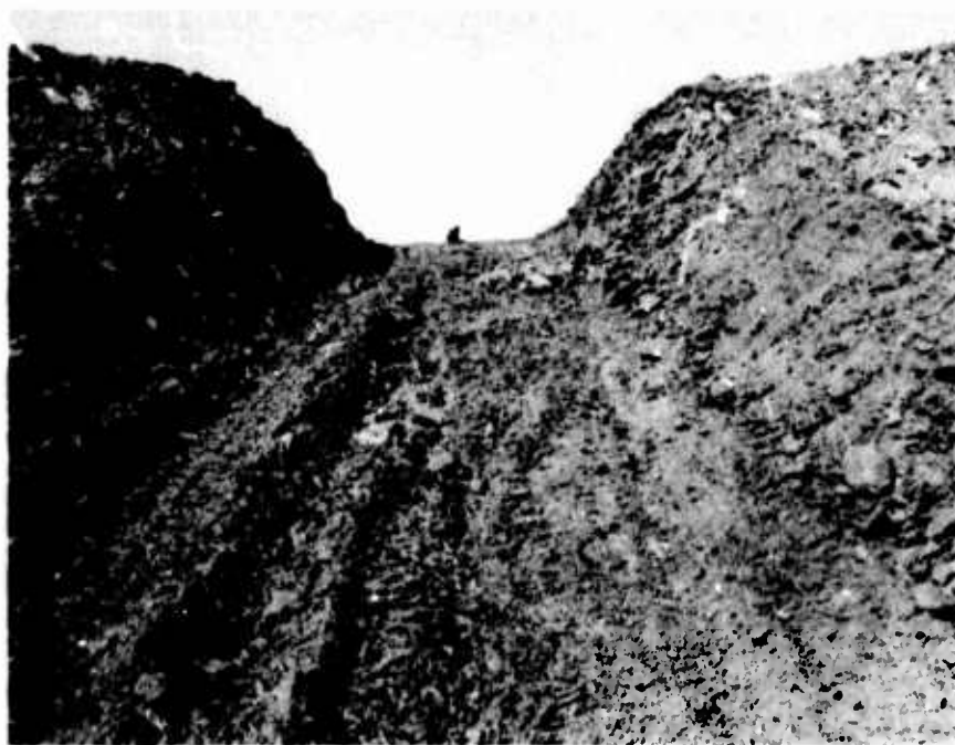
Figure 3.9 Entrance to crater IIA-3 as constructed by D9 tractor.
