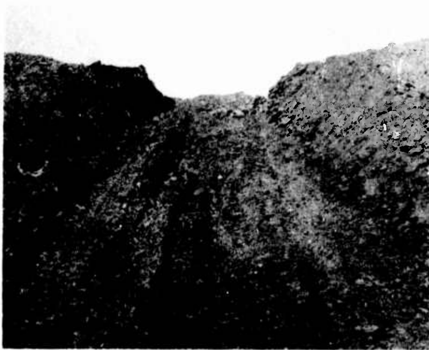
Figure 3.10 Exit from crater IIA-3 as constructed by D9 tractor.
