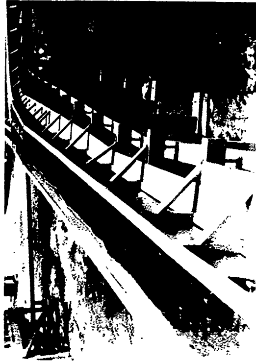
Looking upstream from sta 294+00 Westwood channel 3500 cfs, right side drain 1260 cfs
