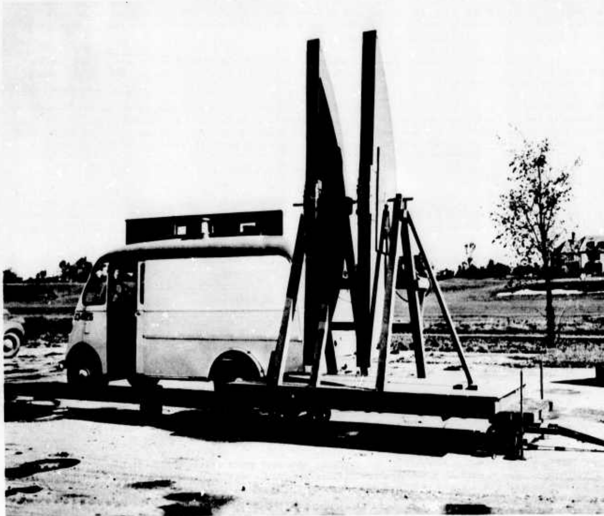
Figure 2.1 Early 3000-MHz Sperry Microwave Glide-Slope System (about 1942)
