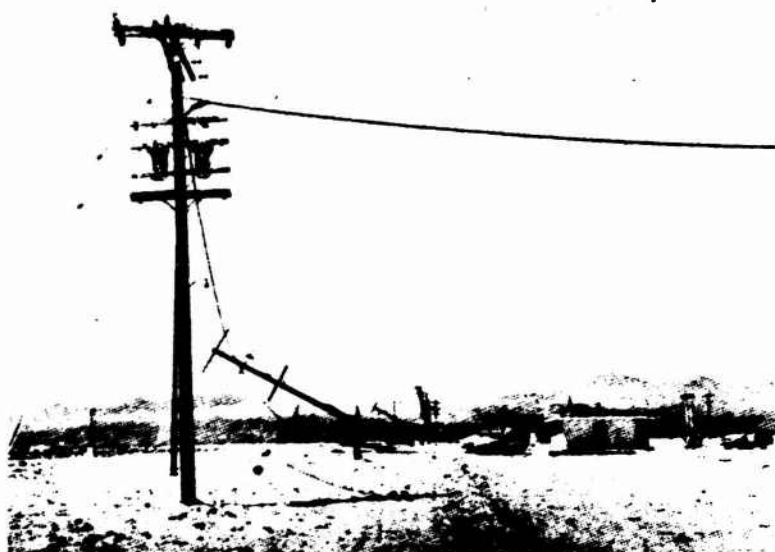
UTILITY POLE DAMAGE AT 5 PSI AT NEVADA PROVING GROUNDS
