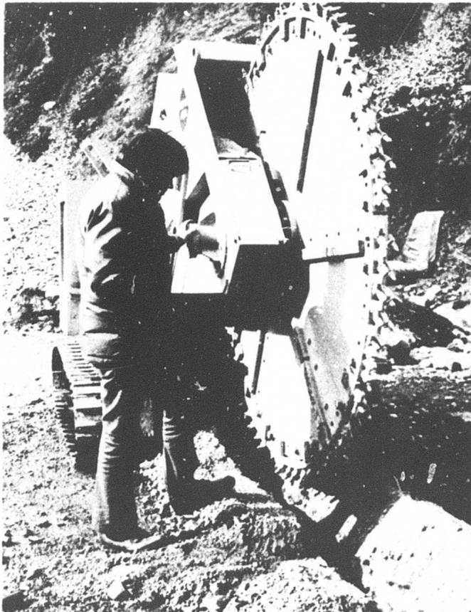
Figure 3. Cutter wheel of Vermeer T-600A. Note radial scouring bars for cleaning cuttings from slot.
