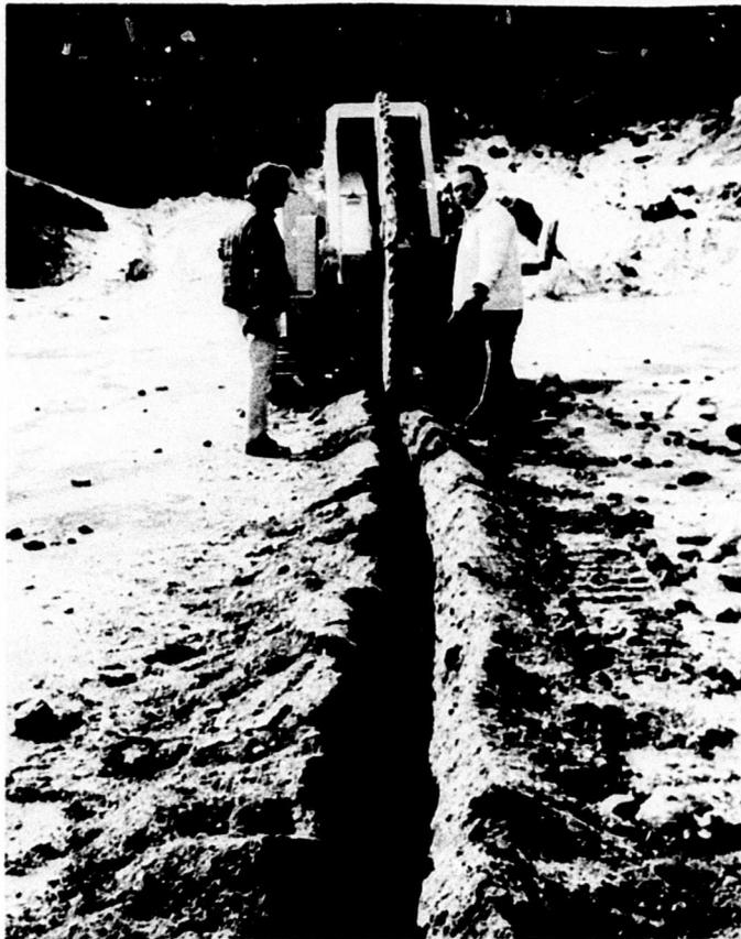
*Figure 8. Vermeer disc saw operating in frozen gravel.*
