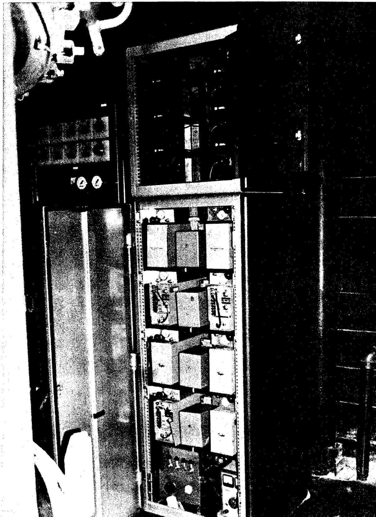
Figure 23. Relative humidity control panel.
