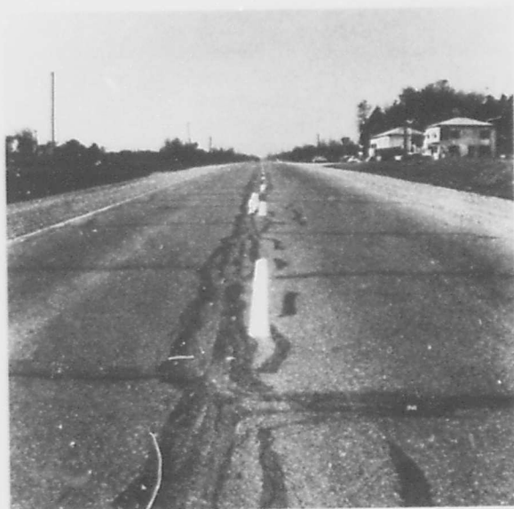
Figure 11. Pavement in Ontario severely affected by low-temperature contraction cracks (25).
