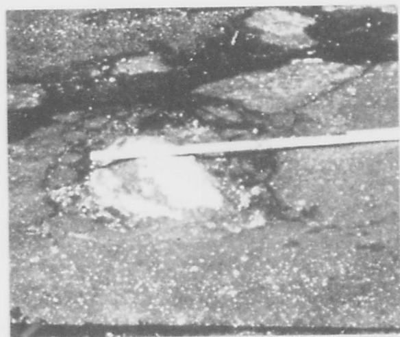
Figure 13. Stone (approx. 9 in.) raised by frost action until it has broken through the pavement surface (28).
