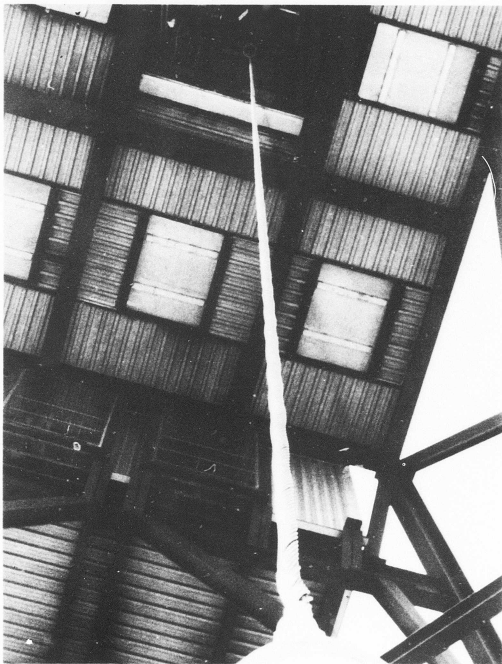
Figure 30. Waves on Cable Assembly.
