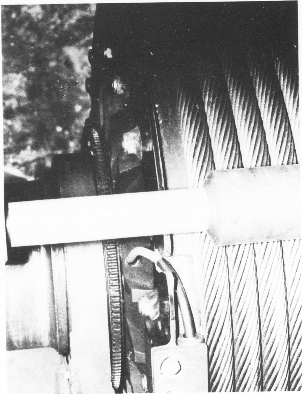
Figure 28. Cable Core Termination on Cargo Hoist.
