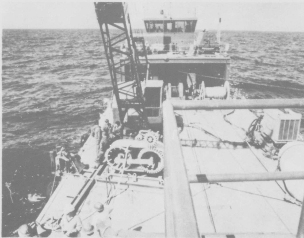
Figure 3.3.3. Equipment setup on warping tug during foundation emplacement cruise.
