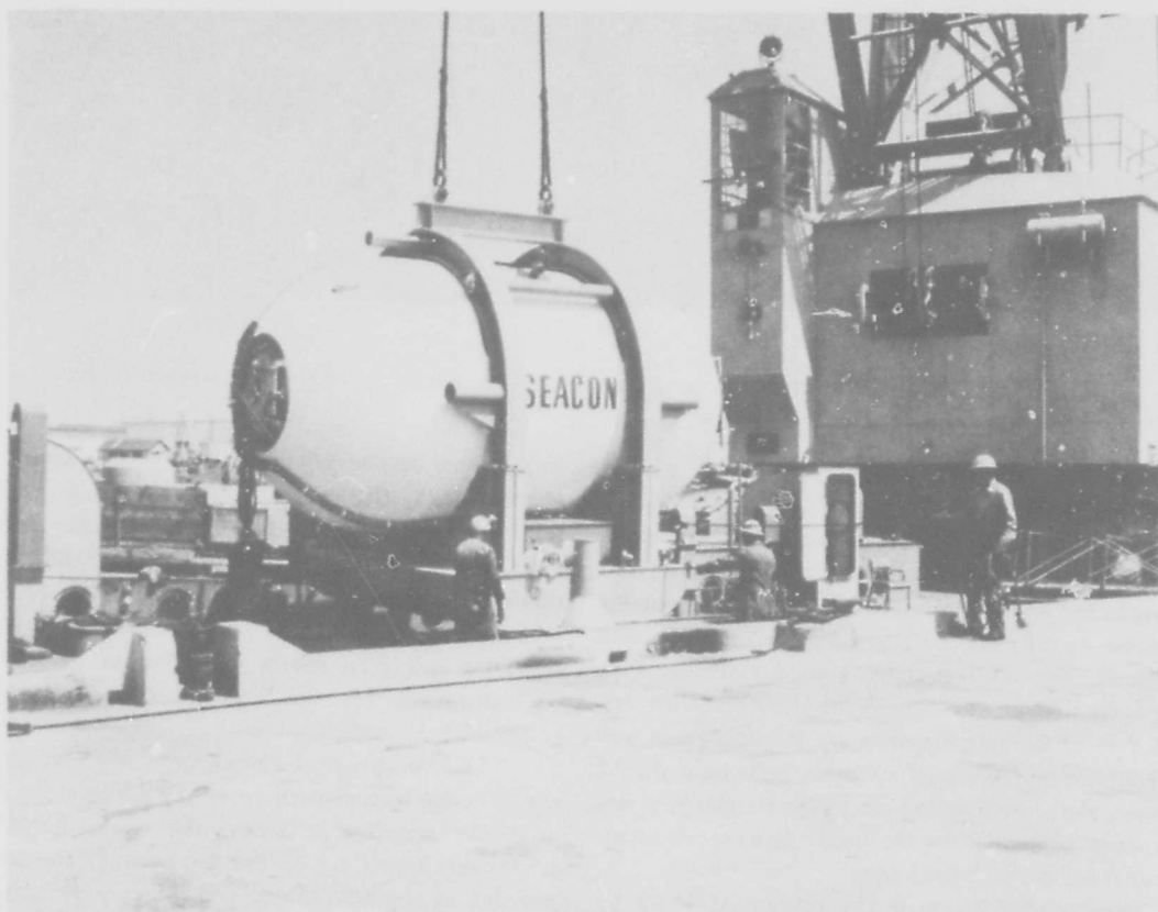
Figure 4.3.1. SEACON, cylindrical concrete structure with 10.1-foot outside diameter, 20-foot overall length, and 9.5-inch wall thickness.
