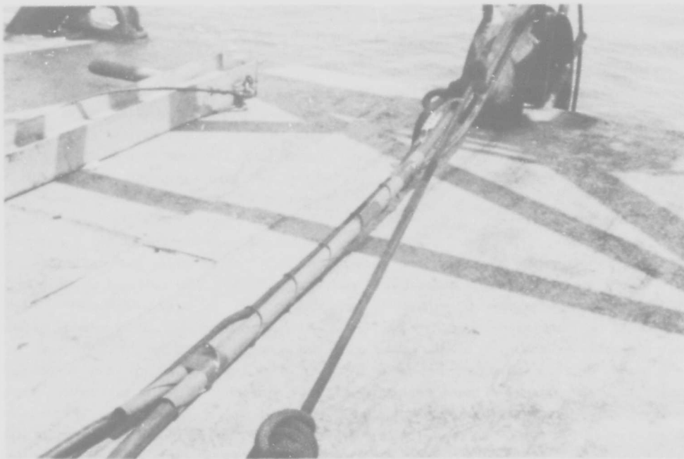
Figure 5.2.9. Paying out cable during SEACON I installation.
