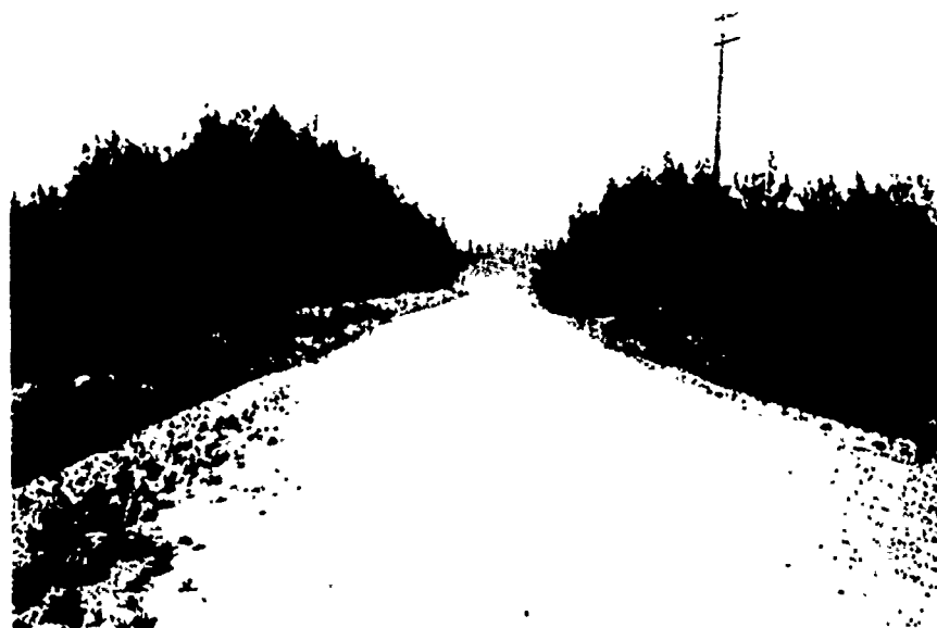
Fig. 35. Well-constructed gravel road.
