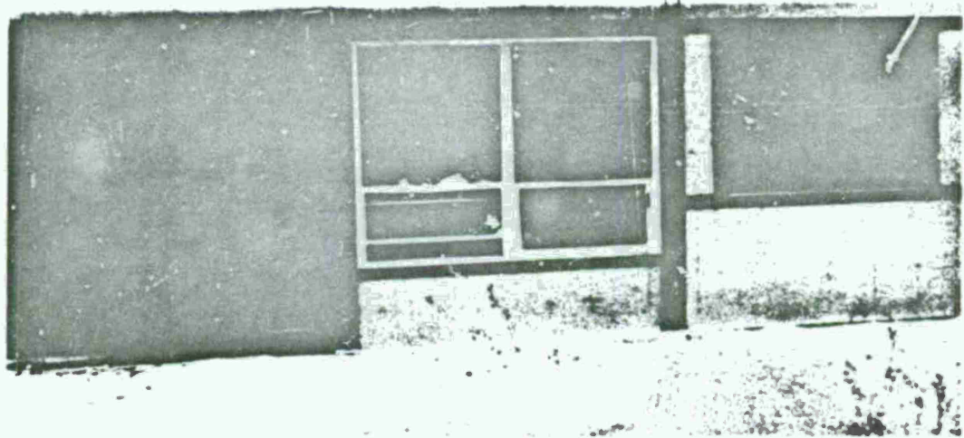
Window Cubes at 1,700 Feet. All window panes were broken out except one.
