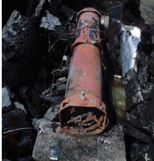
Figure 6 MACS charge after plant fire
