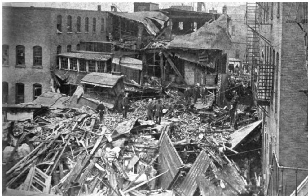
Figure 1 Boiler explosion at Hays Manufacturing Co., Erie, Pa
