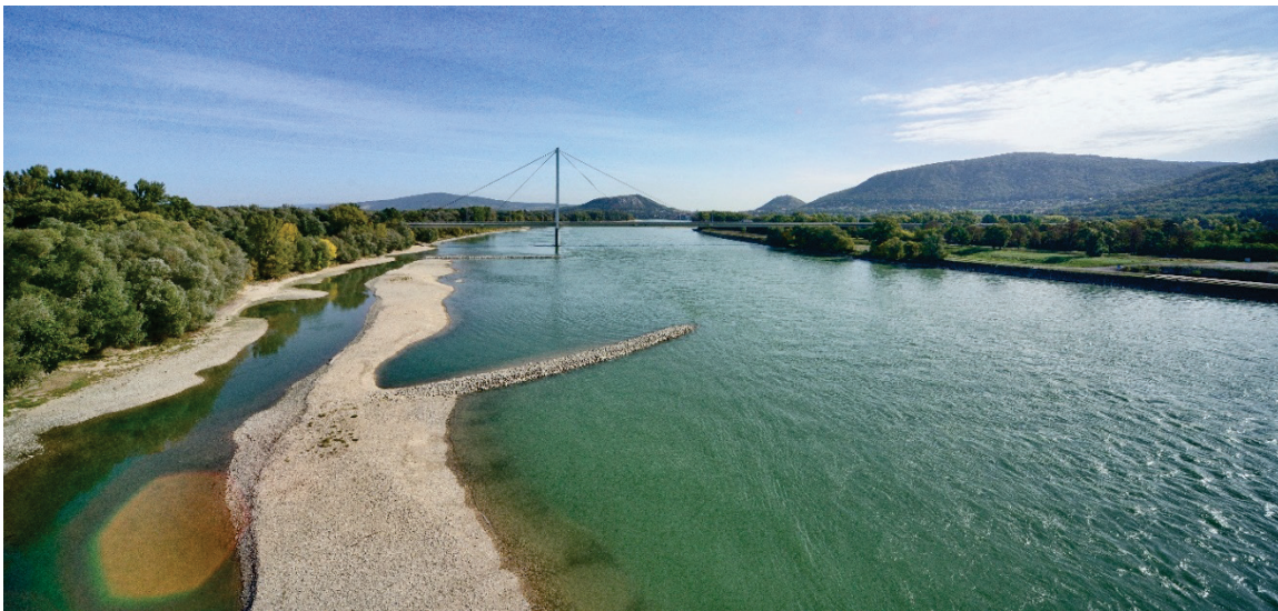
Figure 13. Optimized groyne field Pilot Project Bad Deutsch- Altenburg, downstream (Photo: Viadonau/Zinner).
