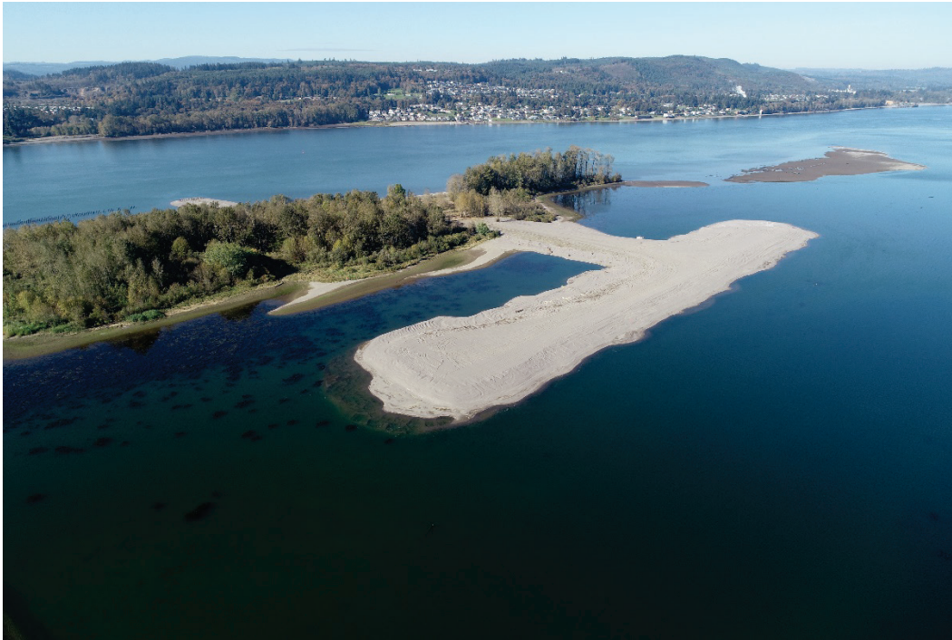
Figure 20. Woodland Island downstream feature constructed in fall 2020 from dredged sediment and subsequent grading for restoring wetland habitats (Photo courtesy Columbia River Estuary Study Taskforce [CREST]).
