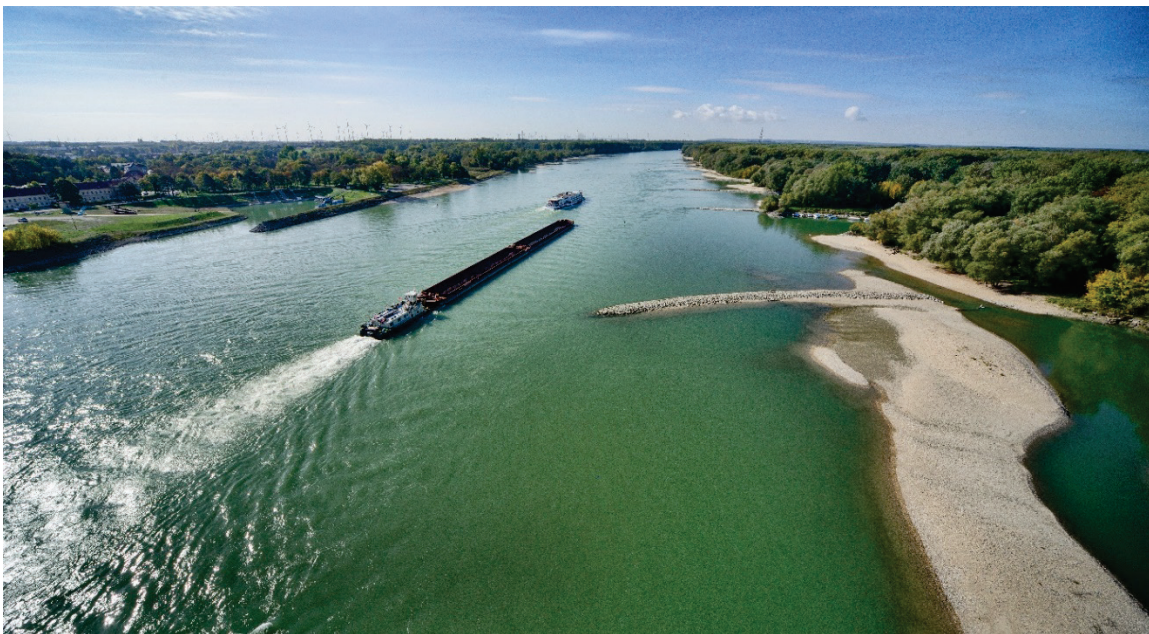
Figure 7. Optimized groyne field Pilot Project Bad Deutsch- Altenburg, upstream (Photo: Viadonau/Zinner).
