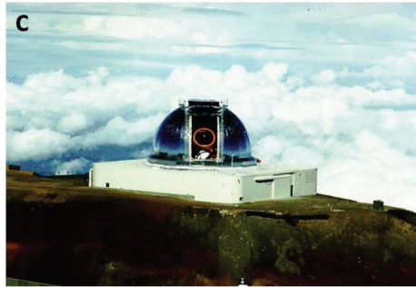
Location: Mauna Kea, Hawaii, USA Aperture: 3.2-meter Focal Ratio: F/38 Field of View: 60 x 60 arc secs Wavelength Range: 0.65-2.55 \mu\text{m} Spectral Resolution: R \sim 100 Focus: Near-IR Spectroscopy
