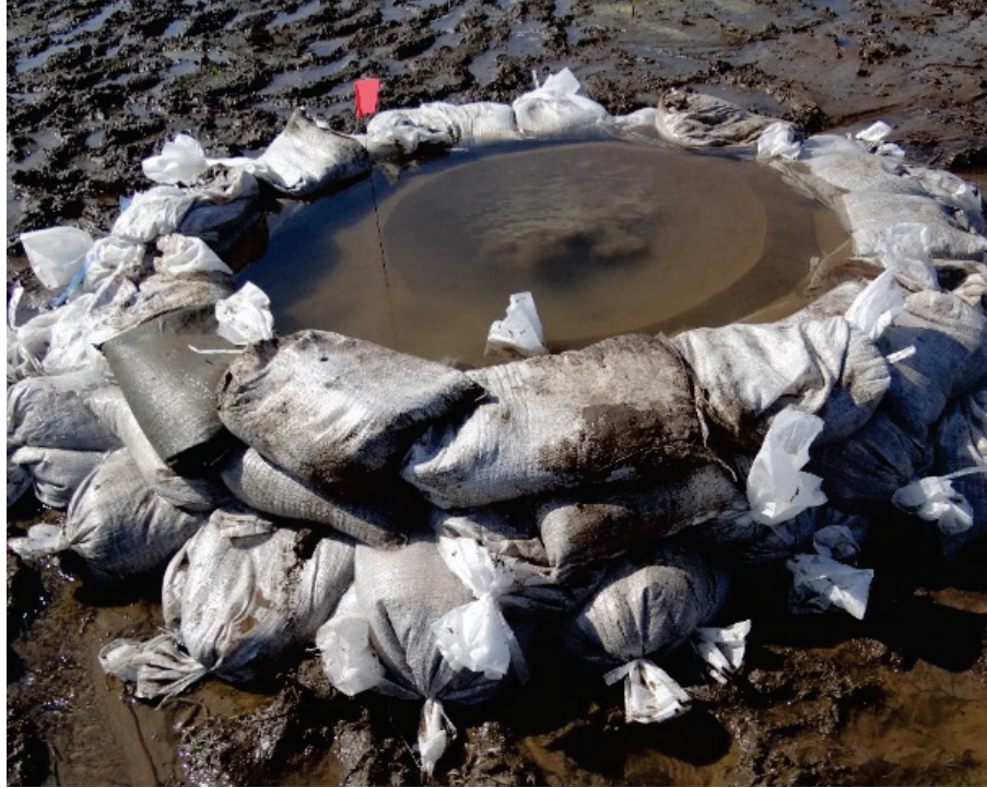
Figure 2. Photograph of typical sandbag ring used to control sand boils.
