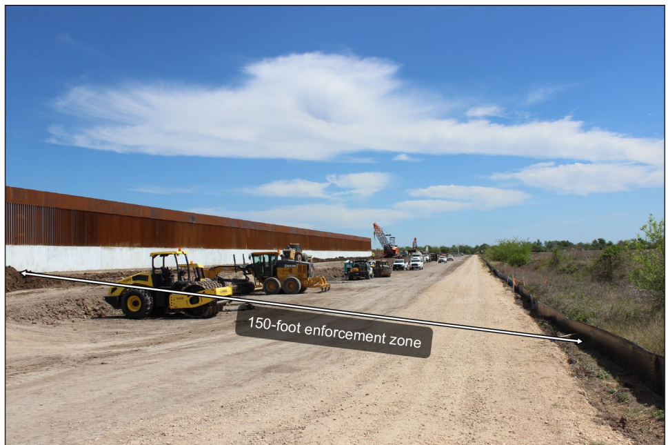
Figure 2: Border Barrier and Enforcement Zone under Construction in Rio Grande Valley Sector
