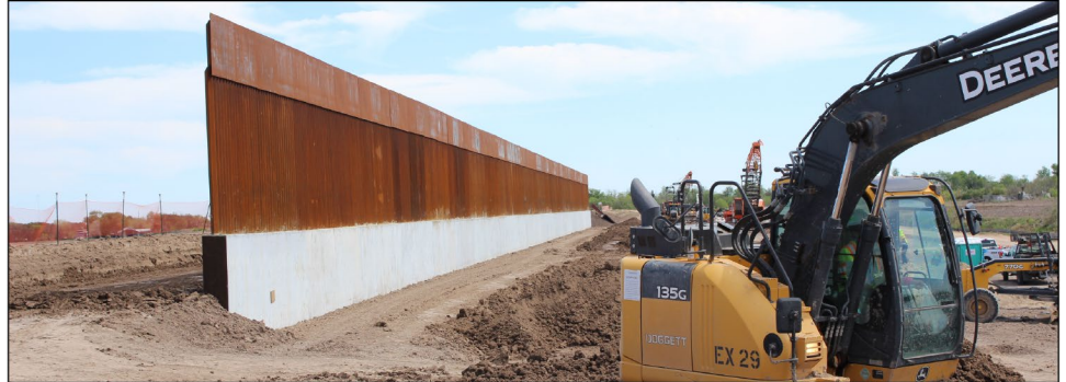
Border Barrier Construction in South Texas
