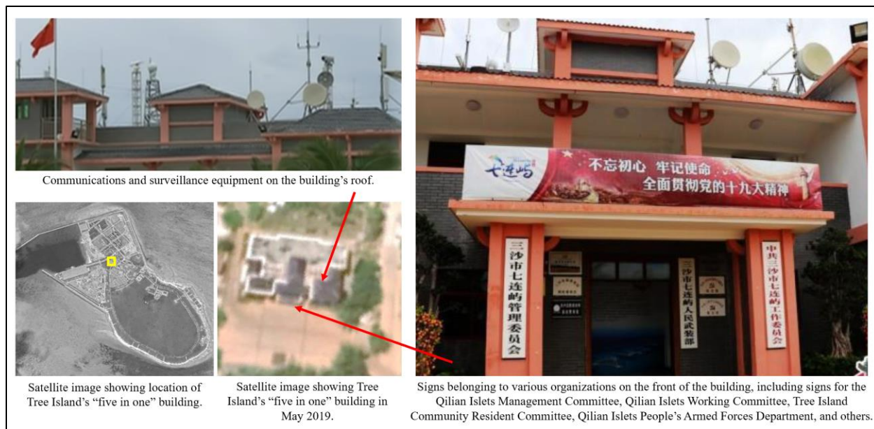
Figure 15. The “five in one” building on Tree Island 298
