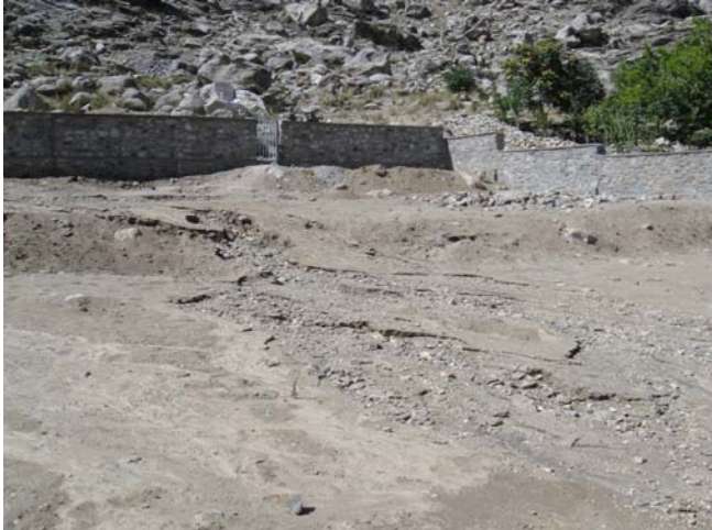
Site Photo 8: View of 2 meter high stone masonry perimeter wall at the rear of the school compound. The significant level of erosion can be seen. The perimeter wall parallel to the slope can be seen on the right. (Photo provided by SIGAR)
