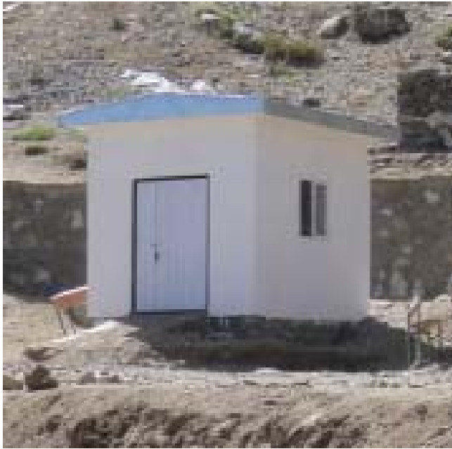
Site Photo 3: View of generator house which lacks proper exhaust venting as required in the statement of work. (Photo provided by SIGAR)
