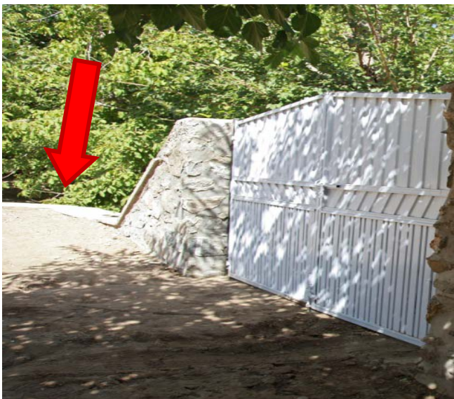
Site Photo 9: The top of the 2 meter perimeter wall can be seen (indicated by red arrow). During the site grading, soil was placed against the perimeter wall, bringing the grade elevation up to the top of the wall in some areas. (Photo provided by SIGAR)
