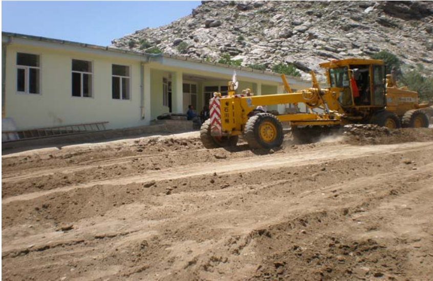
Site Photo 6: View of grader attempting to level the ground in front of the school house in mid- July. This grading improved, but did not solve, the ground erosion problem because there was no follow-up compaction of the soil. (Photo provided by Kapisa PRT)
