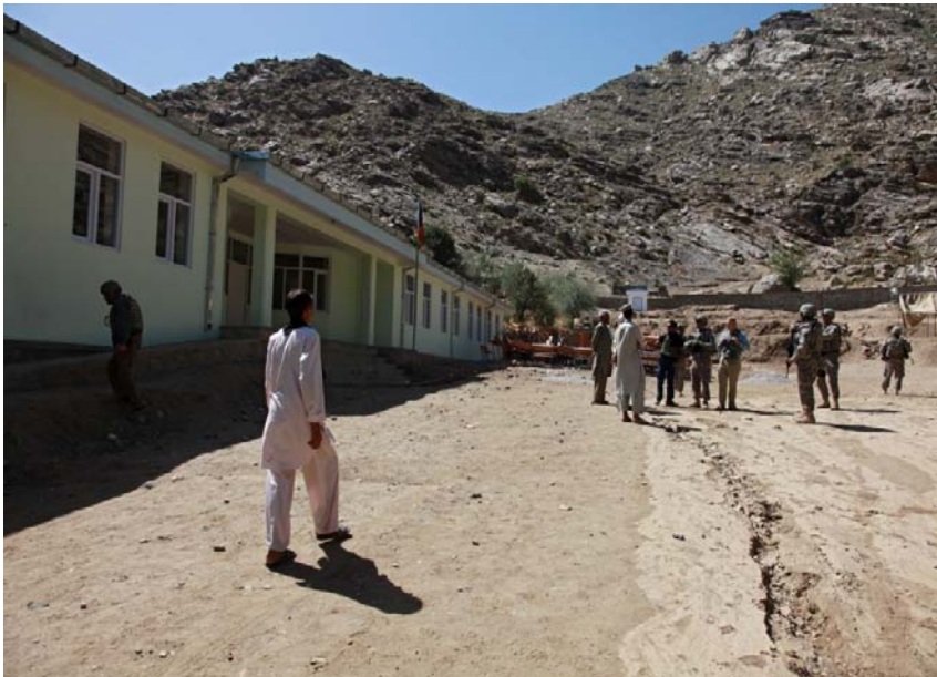
Site Photo 7: View of school grounds less than one month after grading work was completed showing signs of site erosion. (Photo provided by Kapisa PRT)
