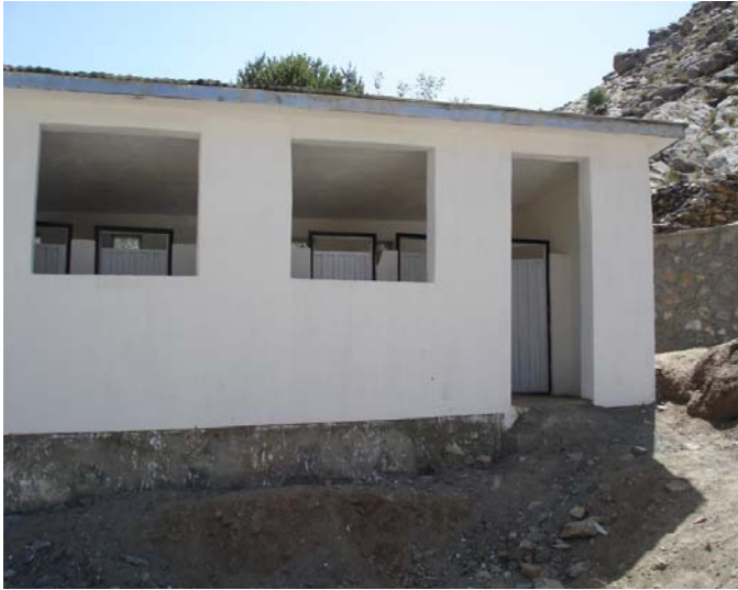
Site photo 2: View of the latrine containing inadequate opening sizes for refuse removal. (Photo provided by SIGAR)
